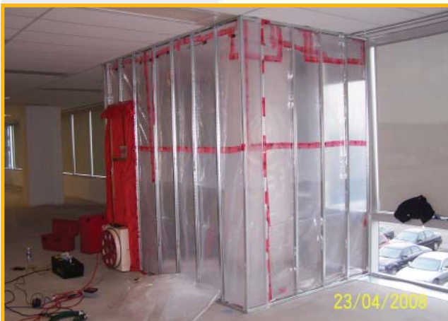
Sealed test chamber on inside of curtain wall.
